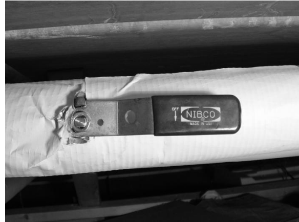
Ball valve in open position
